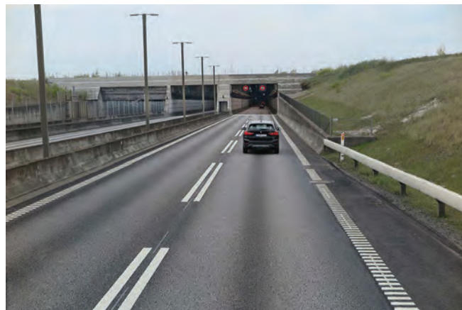
Our return coach journey to Denmark – about to transition from bridge to tunnel on Pepper Islet. The middle portal houses the eastbound road carriageway; the wider portal for the two rail tracks can be seen to the left hand side
